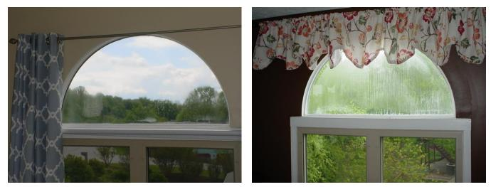
• Moisture has condensed in the space between panes in several windows. This failure of the seal between the panes can affect the insulating value and the clarity of the windows.
