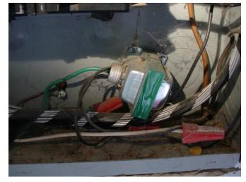
• **Safety Issue:** Multiple neutral wires are connected to several neutral bar terminals. For the most reliable wire connection that offers the least risk of overheating, each neutral wire should connect to a terminal that is not used for another conductor.
