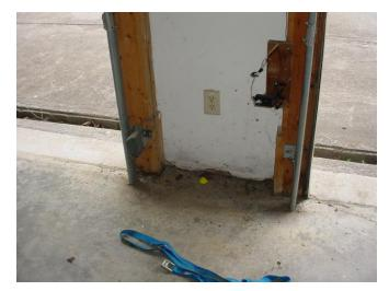
• **Repair:** The center rail has separated from the bottom panel of the front garage door.
